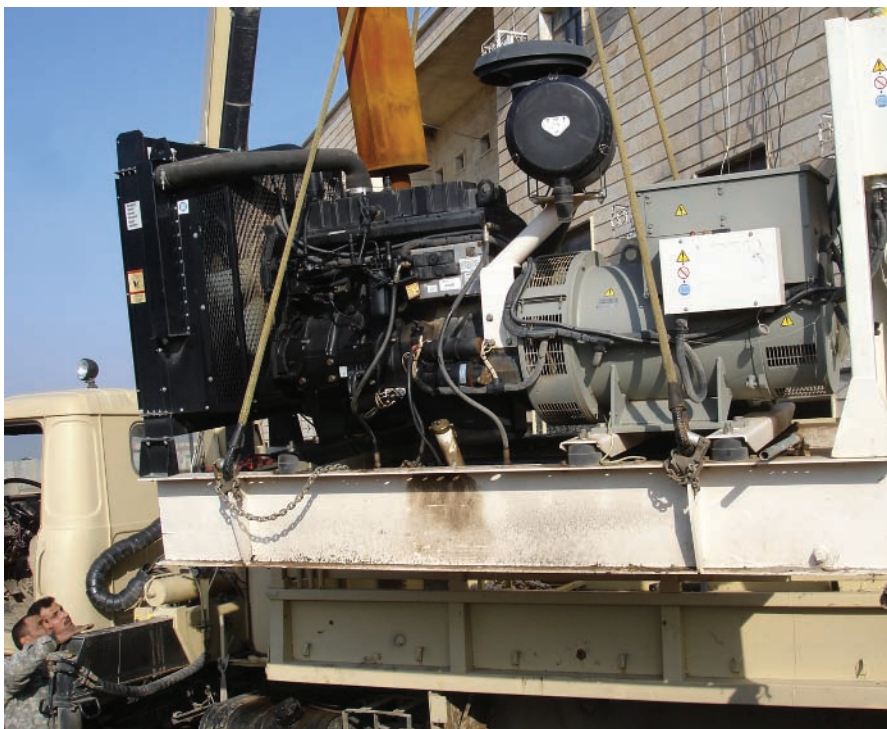
A Kraz 7.5-ton truck with Inman crane and Iraqi operator is used to remove a generator for maintenance.
